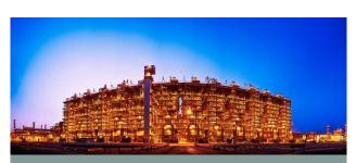
The Sadara Mixed Feed Cracker (MFC) is the only one of its kind in Saudi Arabia, cracking both ethane gas and naphtha liquid simultaneously. It enables Sadara to produce a range of high value plastic and intermediate chemical products.
